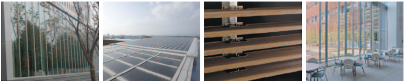
Fig. 4-5: Effective utilization of natural energies. From left to right: Photocatalyst-coated glass watering system, solar panels, wooden louvers and automatic blinds control system.
