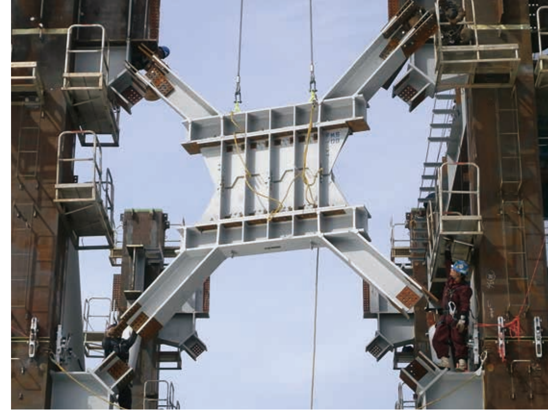
FMS alloy seismic damper being integrated into the JP Tower Nagoya
