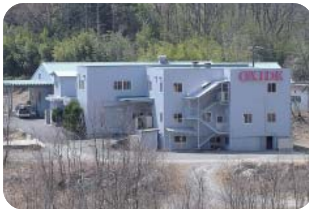
OXIDE Corporation's new building at Takekawa, Hokuto City, Yamanashi Pref.
