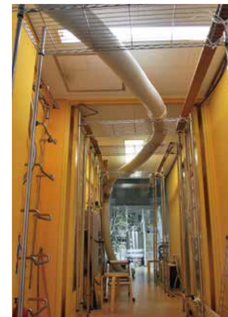
Laying a pipe for liquid nitrogen over steel racks
